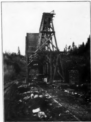
End View of Loading Bunkers
